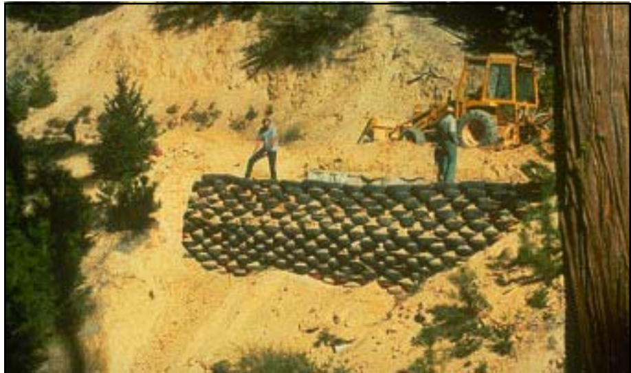
Photo 11.11 A tire-faced, mechanically stabilized earth (MSE) retaining wall, with layers of geotextile reinforcement, being used to gain road width in a fill failure area. MSE (reinforced soil) structures are often the least expensive retaining structure available. Welded wire MSE walls are also commonly used.
