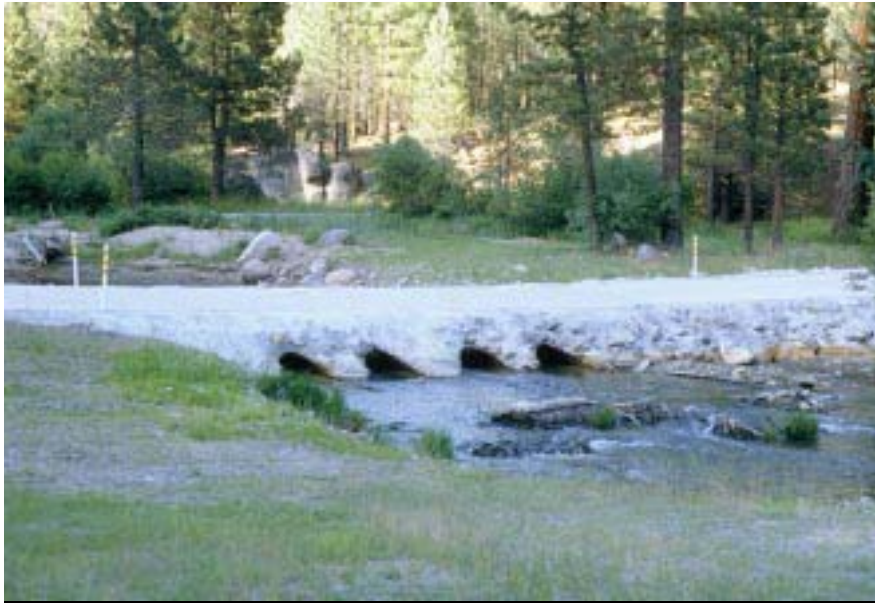
Photo 9.2 A vented ford, using multiple culvert pipes to handle low flows through the pipes, yet allow major flows and debris to overtop the entire structure.
