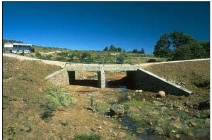
Photo 8.3 Install masonry/concrete box or metal culverts with a large enough size (capacity) to safely pass the anticipated design flow (typically a 20- to 50-year recurrence event), based upon hydrological analysis. Use headwalls and wingwalls whenever possible.
