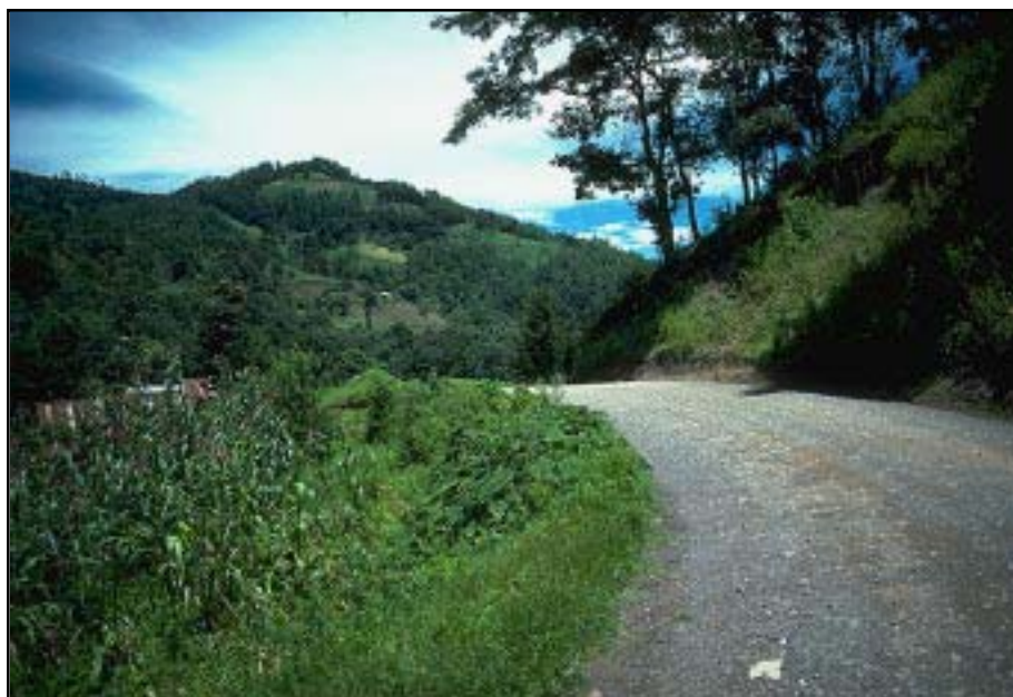
Photo 2.5 A well designed, “minimum impact” road that has an appropriate standard for its use, good drainage, and stable slopes.
