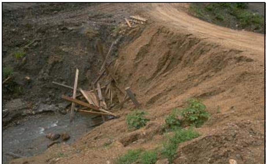
Photo 11.4 Avoid loose, over-steep fill slopes (steeper than 1 1/5:1), particularly along streams and at drainage crossings.
