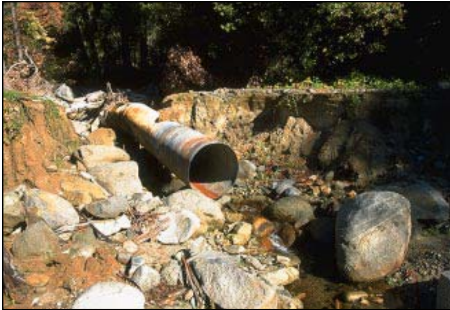
Photo 8.2 A culvert failure caused by insufficient flow capacity or inadequate pipe size to pass the debris (boulders) moving through the drainage.
