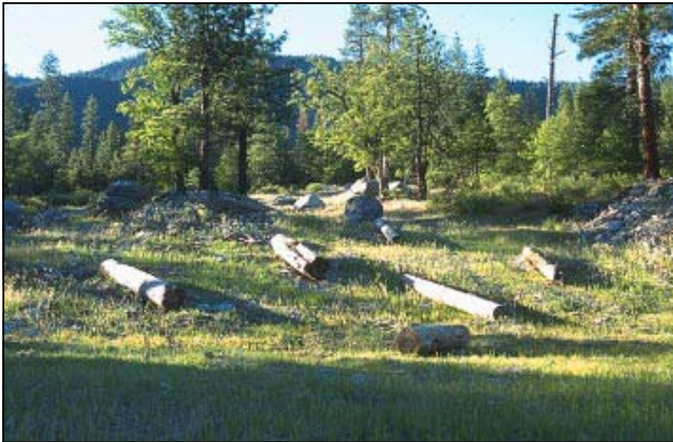
Photo 12.12 A reclaimed and revegetated borrow site. Reshape, drain, plant vegetation, and rehabilitate borrow pits and quarries once the usable materials are removed and use of the area is completed.
